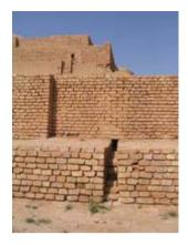
The water of the river Karkheh was not among the most healthy, so it was necessary to clean it before it could be used at the shrine. This picture shows the installation in which the water was refined. It was led through several basins; this picture shows the first and largest.
